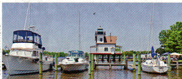
The newly-restored Roanoke River Lighthouse
